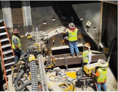
MTBM would encounter mixed ground that could lead to a loss of face pressure and, in turn, result in serious ground control issues. Working beneath the rail lines added extra pressure.
