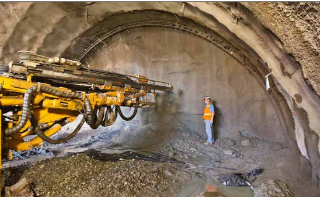
Probe drilling ahead from stabilized face – Caldecott Fourth Bore Tunnel
