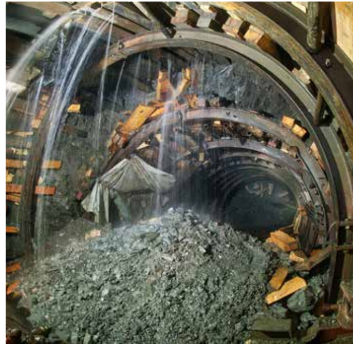
Difficult tunnel mapping conditions in bad ground – New Irvington Tunnel
