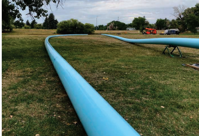
Figure 5 – Lay down area for HDD casing
