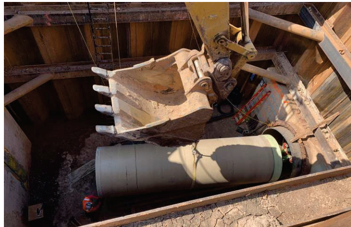
Figure 2 – Example of microtunnel launch pit
