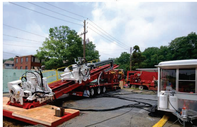
Figure 3 – Directional drilling process (top) and drill rig and control trailer (bottom)
