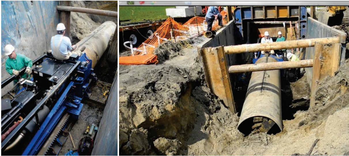
Figure 1 – Pipe jacking launching pit with steel casing
