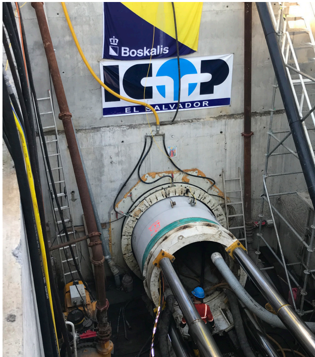
Microtunnel Entry Pit Area
