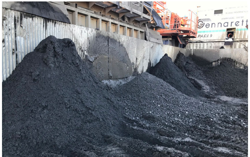
Cuttings piles showing mix of sand piles (separated by gravel), with fines separated out in background.
