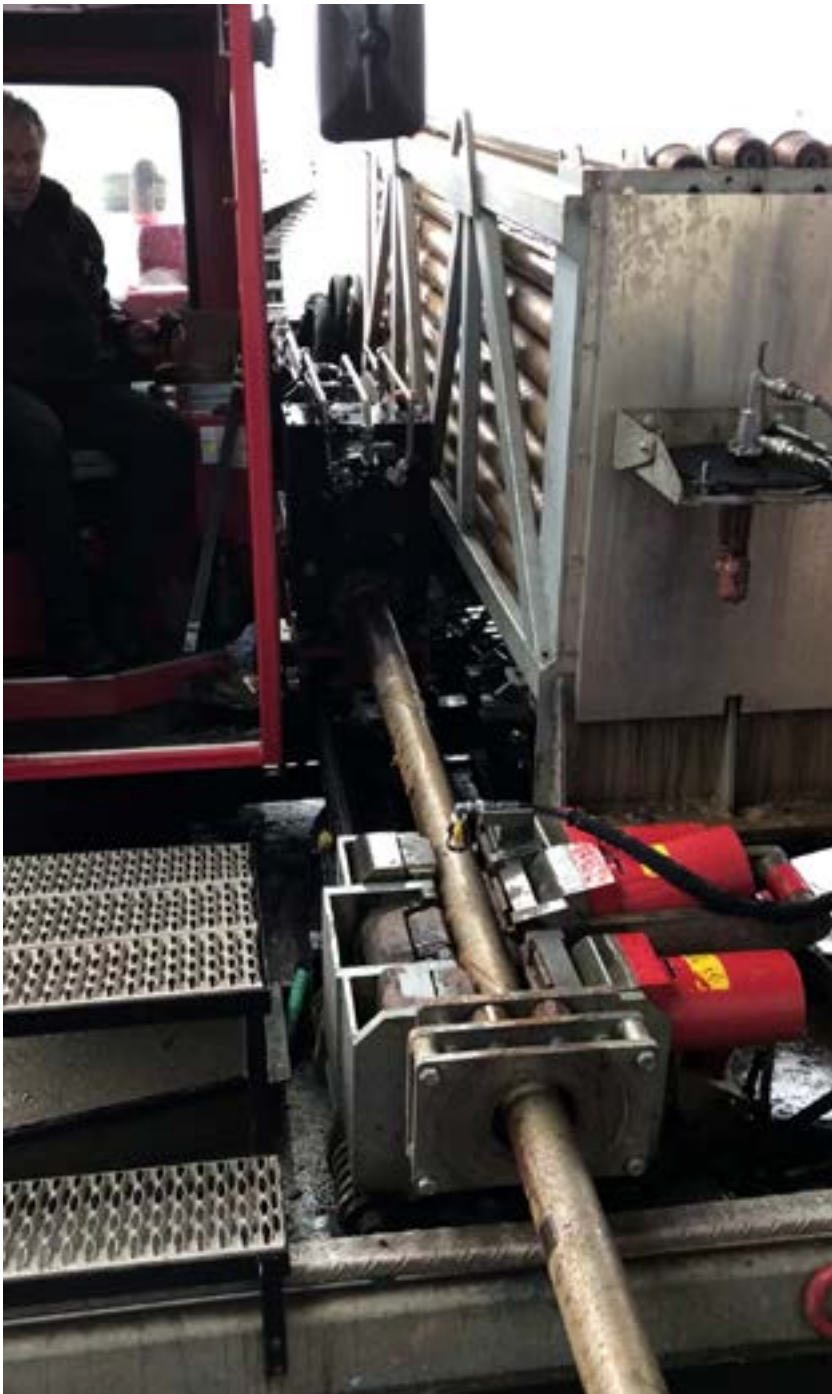
Figure 2. Prime P-80 drill turning dual rods. (Photo courtesy of Ellingson Companies.)
