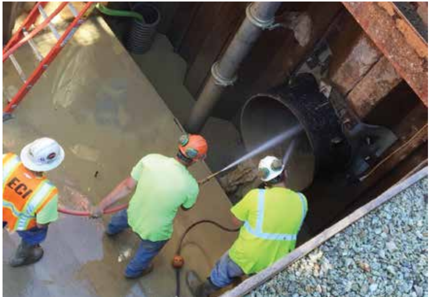
Cleaning the 42-inch casing
