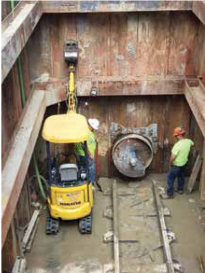
Auger bore through 42-inch casing
