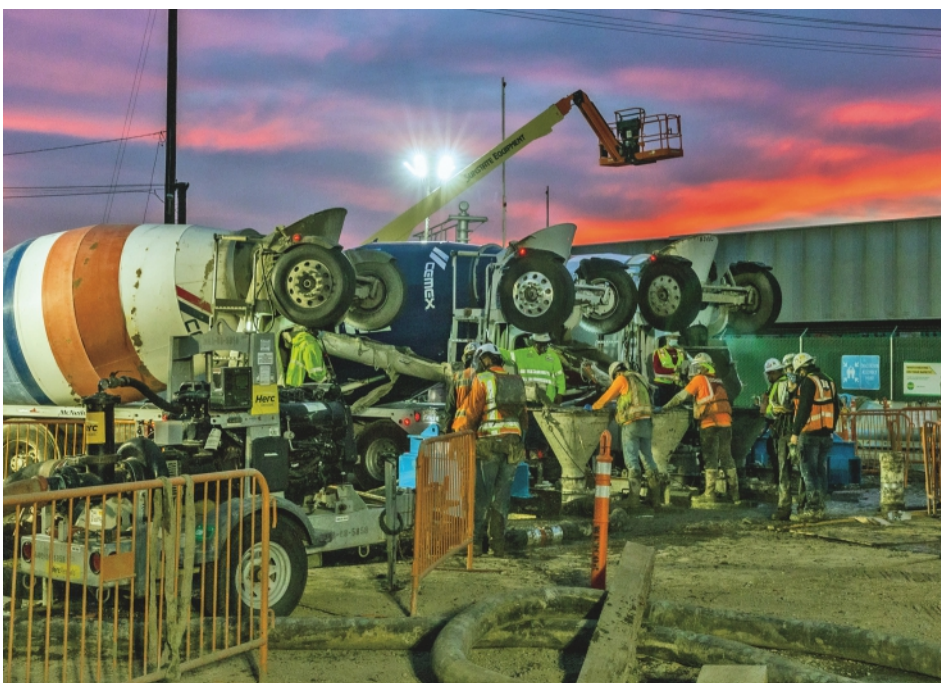
Primary panel concrete placement with simultaneous excavation in background
