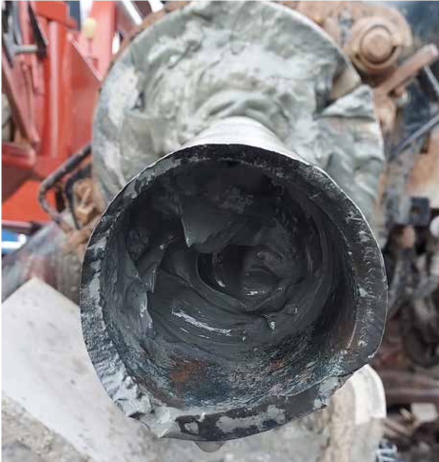
Drill fluid is a key component of HDD project success
