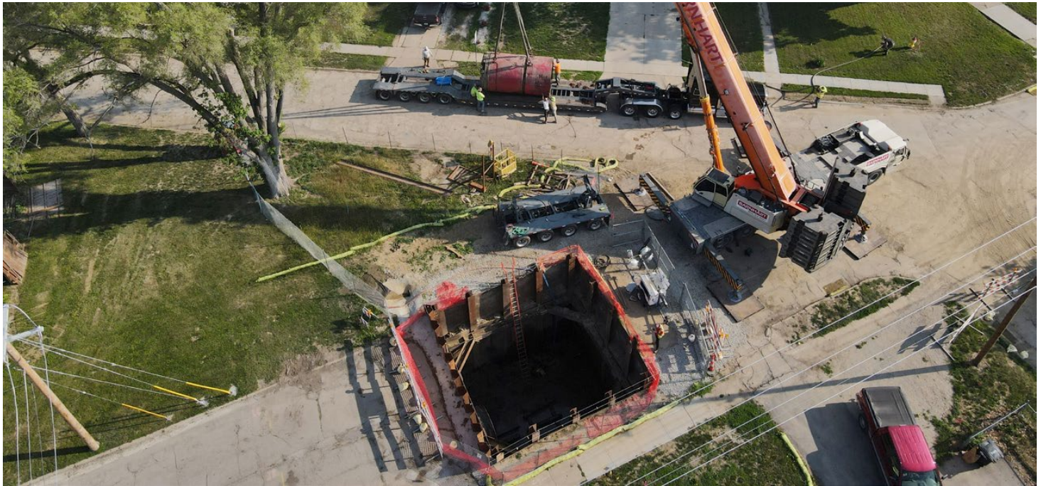
1300 Linear feet, 96-inch microtunnel crossing within a residential area
