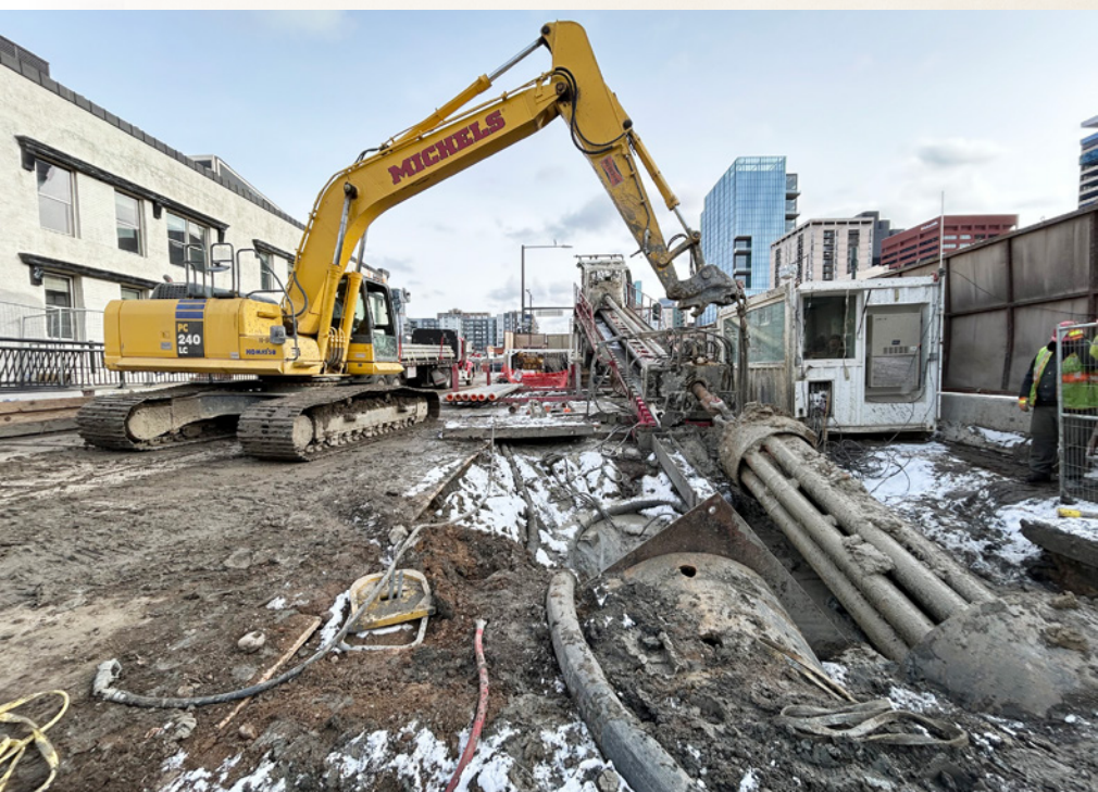
Pullback completed in only two shifts
