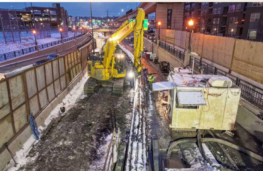
Duct bundle pullback completed during late spring snowstorms
