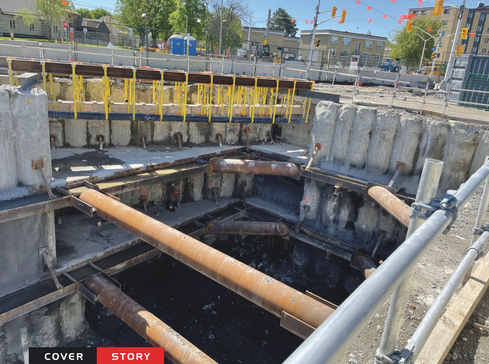
Zone 13a utility adit with levels 1 and 2 framing
