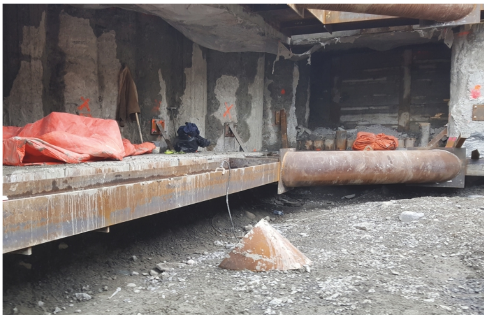
Zone 13a utility adit with level 1 and 2 diaphragm slabs installed
