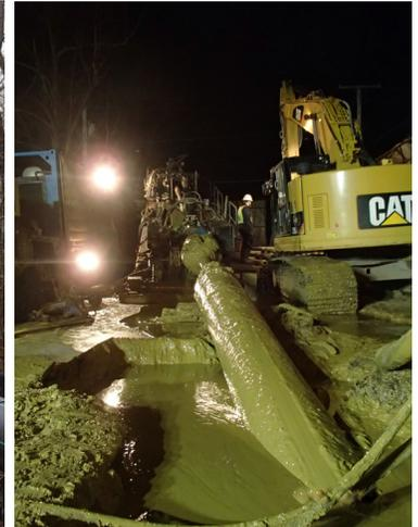
Brierley Associates led the HDD design team that was challenged by subsurface ground conditions consisting of deep, very soft soils. To mitigate the potential of inadvertent drill fluid losses, a bore depth of over 100-ft deep below river bottom, was chosen. Through our design analysis we selected 24-in diameter, DR-7 HDPE that was capable of withstanding the installation forces.
