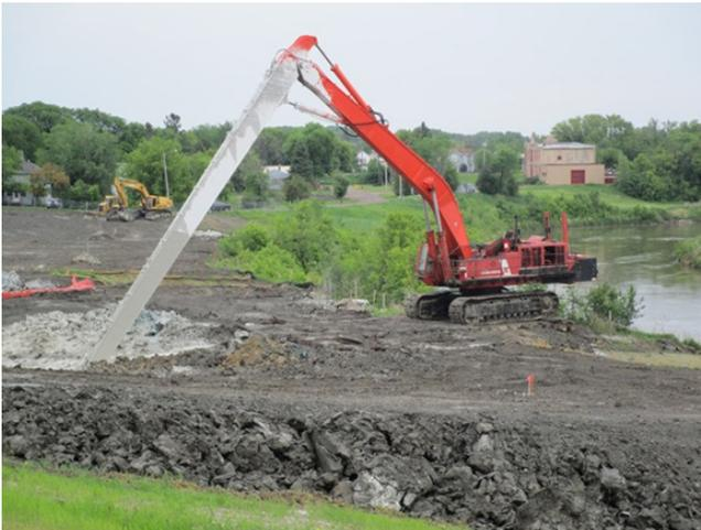
*“Long Stick” excavator used to construct the CB shear walls.*
