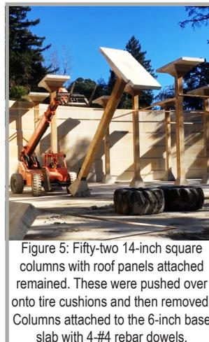
Figure 5: Fifty-two 14-inch square columns with roof panels attached remained. These were pushed over onto tire cushions and then removed. Columns attached to the 6-inch base slab with 4-#4 rebar dowels.
