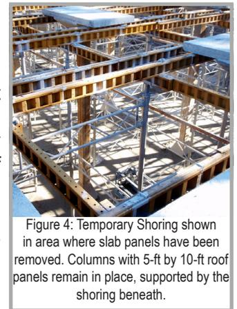
Figure 4: Temporary Shoring shown in area where slab panels have been removed. Columns with 5-ft by 10-ft roof panels remain in place, supported by the shoring beneath.
