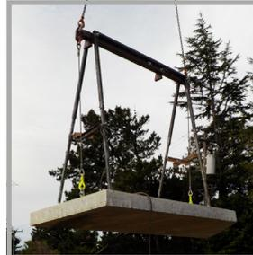
Figure 3: Typical 5-ft by 10-ft panel being removed. Work was eased by the four adjustable stop post prongs extending from the spreader that allowed the use of only two Monkey Fist removable concrete anchors.
