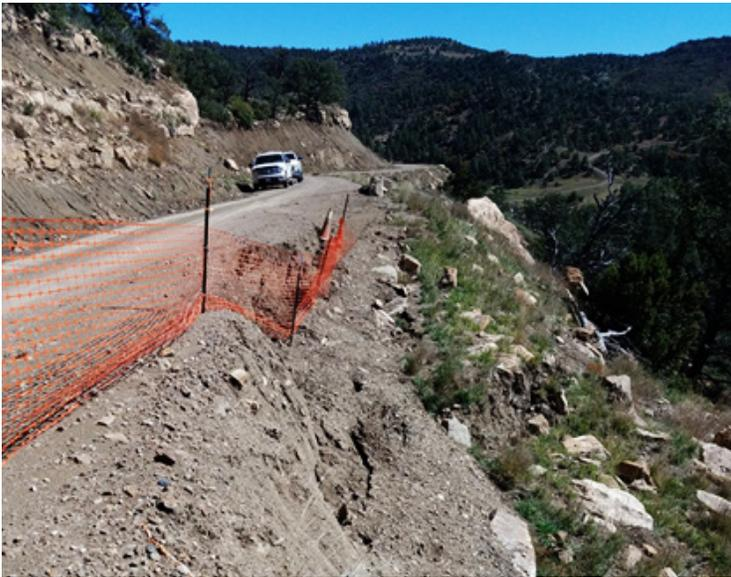
Regionally, during the first six months of 2017, total precipitation was about 50% more than average. Then, in August 2017 a sudden ground movement occurred which disrupted the use of an unpaved access road that hugs the side of a canyon. The landslide was approximately 200-ft long and somewhat parallel to the roadway, with a more active center portion about 100- to 150-ft wide.
