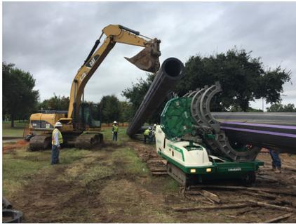
recommendations during the geotechnical investigation; design of the horizontal directional drilling (HDD) path and pipe calculations; a geotechnical baseline report (GBR); and construction management assistance. Components of this project included: 8-, 12-, 24- and 32-in diameter pipelines constructed by conventional open cut methods and trenchless technology.
