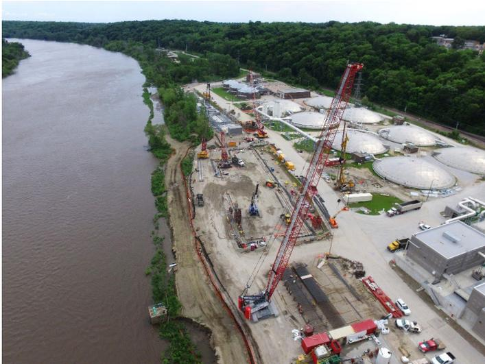
Aerial photo of MRWRRF during installation of the CCB diaphragm wall.
