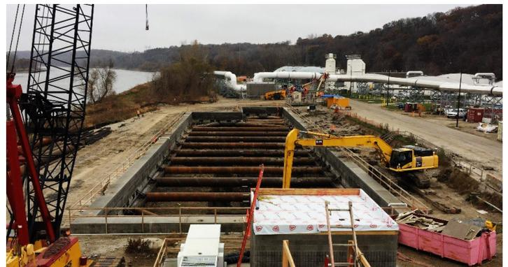
Excavation of CCB after installation of first level of internal bracing.
