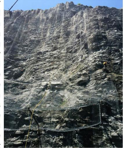
of the connection between canopy and drape was to create a “slot”, which falling rock would be retained within the system and would not exit the netting limits. Our design team opted for the rockfall canopy arrangement, which could be adapted to the field conditions and not restrict construction access by the tunneling crews.
