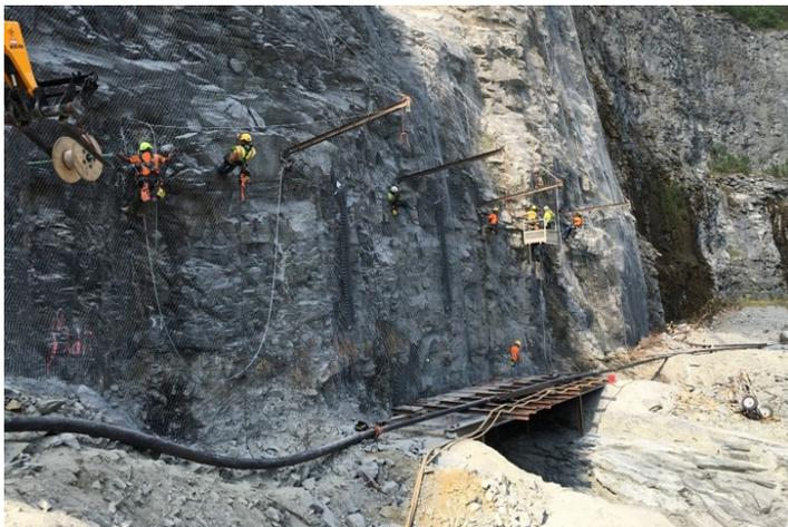
The netted segment of slope above the tunnel portal is about 315-ft high and 365-ft long. G65/3mm Tecco® Mesh by Geobrugg was selected for temporary and permanent rockfall mitigation purposes. The netting is supported at the crest by a series of ¾-in diameter wire rope anchors and a top rope. The temporary draped netting was locally tied into the canopy system. The intent
